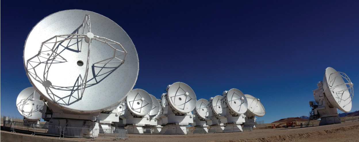
ALMA's 16-antenna Atacama Compact Array, or ACA, enhances imaging fidelity for extended astronomical sources. Credit: ALMA(ESO/NAOJ/NRAO)
